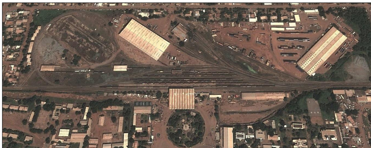
Figure 5-3: Ouagadougou railway facility
