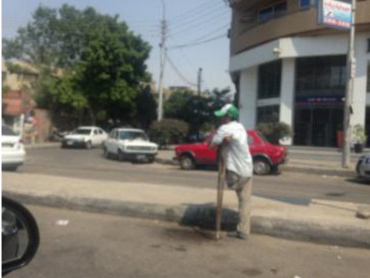
Figure 38: No dropped kerbs/ramps for disabled people to cross the roads
